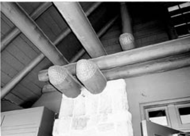
The Arts and Crafts movement is reflected in the logs and stone masonry of Old Faithful's Upper Hamilton Store. NPS photo.
