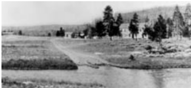
Figure 10. Late 1880s view of the Marshall/Firehole Hotel (courtesy Yellowstone National Park Archives).
