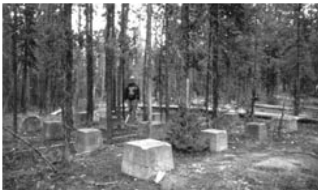
Figure 16. Concrete supports for the Fountain Hotel's water tower (NPS-Midwest Archeological Center Archives).
