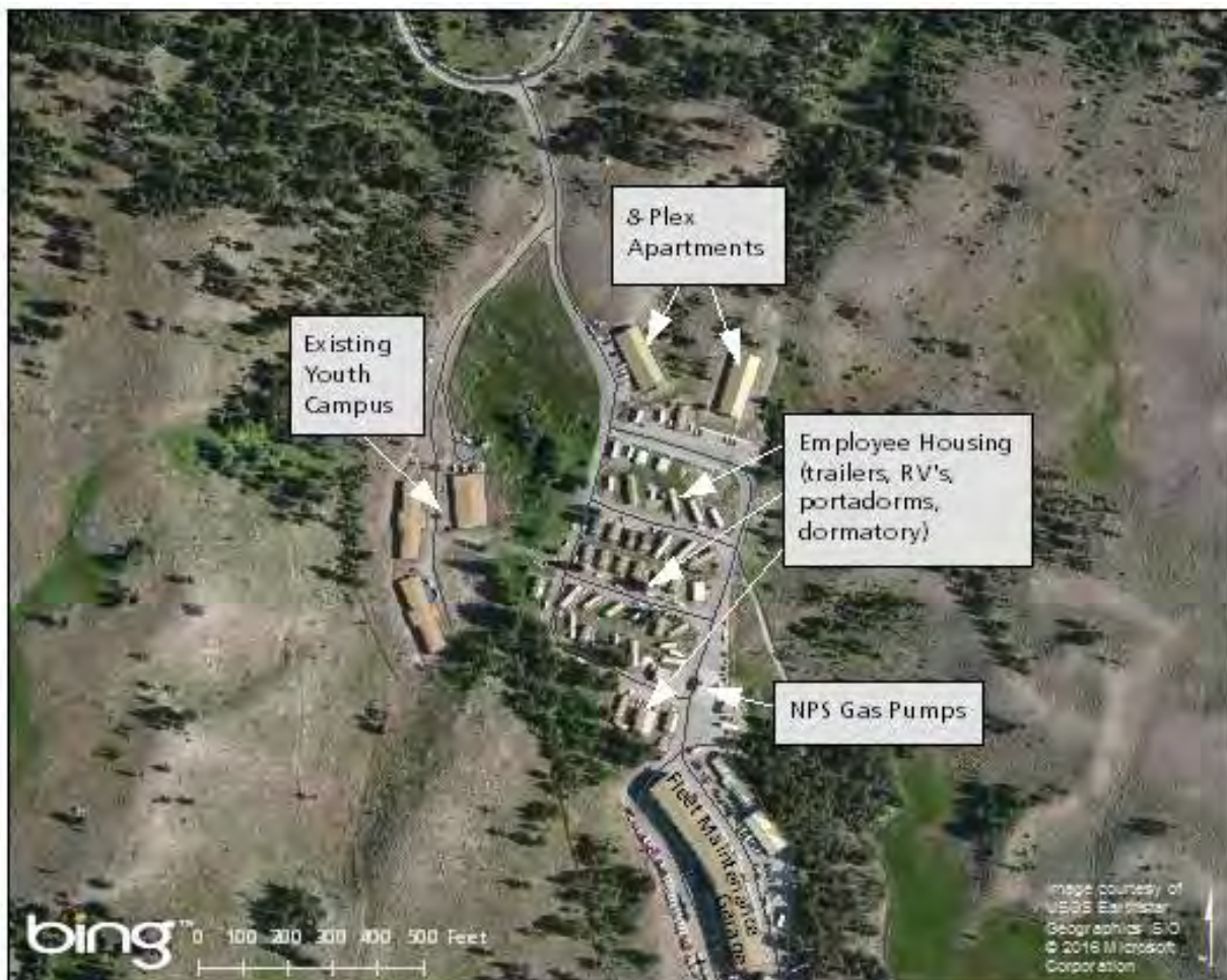
Figure 1: Existing Youth Conservation Corps (YCC) Campus
