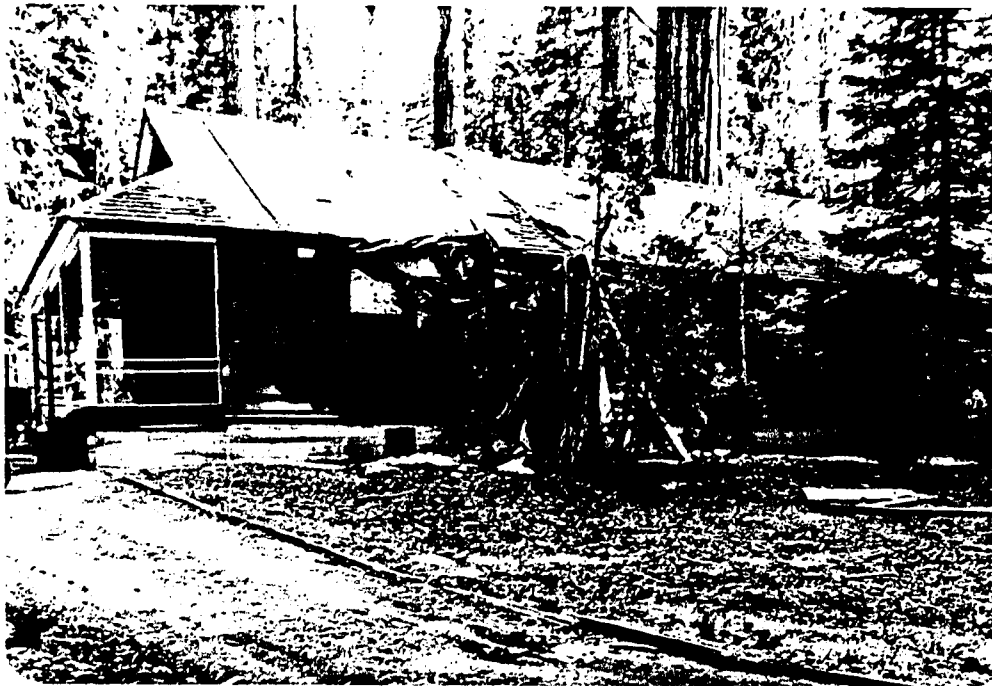
Figure 2: The west end of the building from the southwest.
