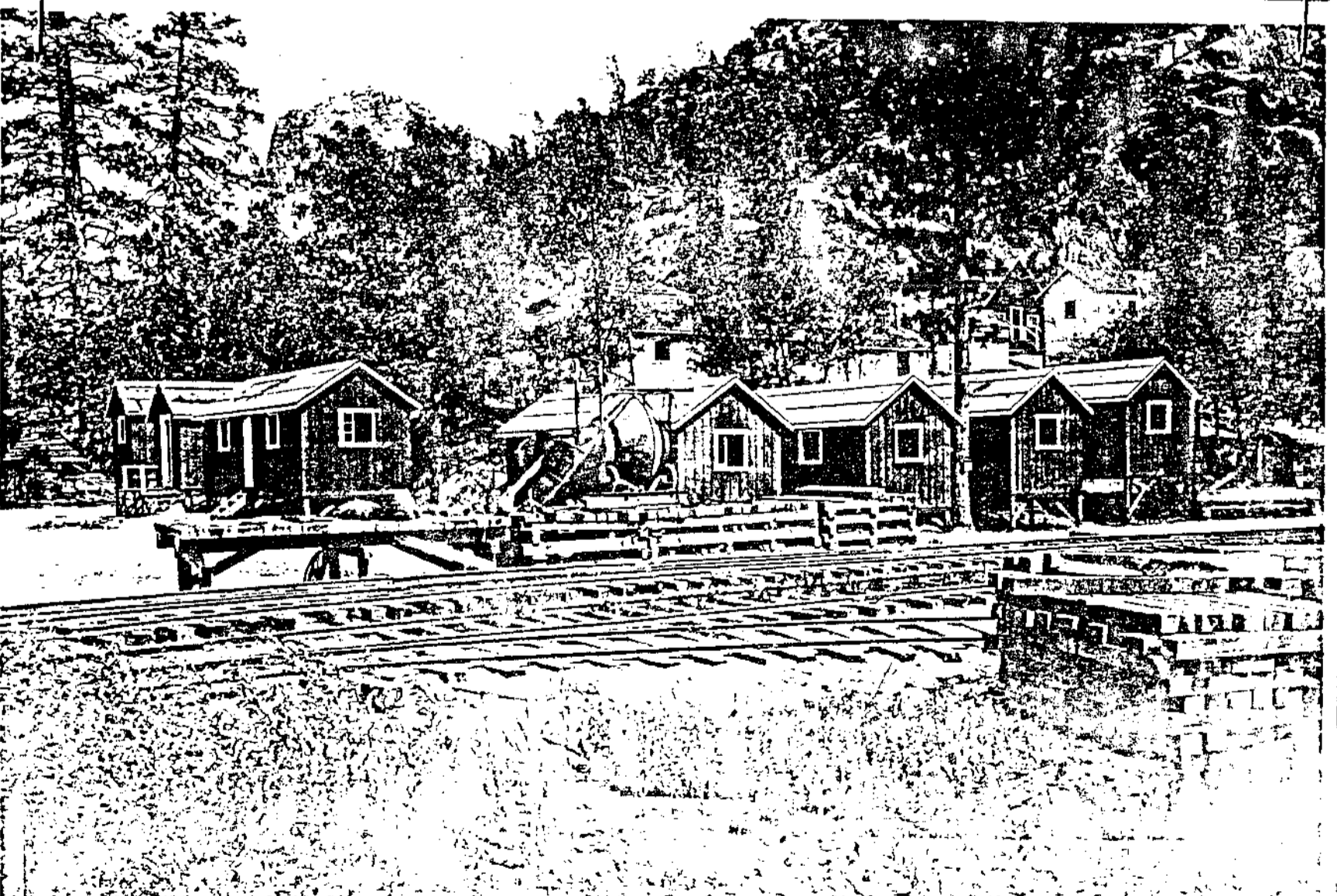
5211 - 8-28-19 H.H. Dam - Portable Bankhouses
