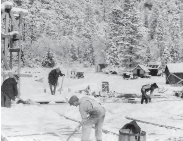
Removing snow from floor slab form work, 1924 (Yosemite Archives).
