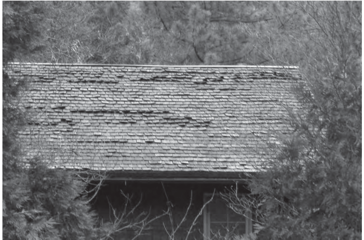
Curling shakes on main central roof, 2006.
