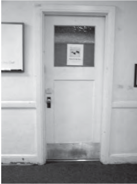
Typical door, second floor hall, 2006.
