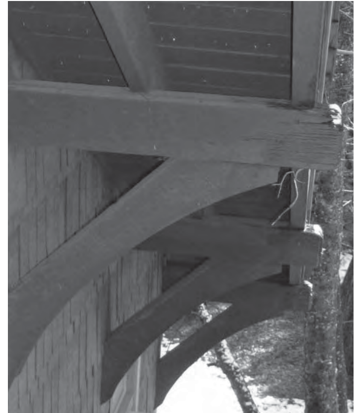
Roof braces, west elevation, 2006.
