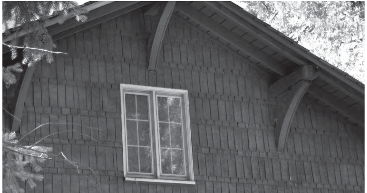
East elevation window attic window, 2006.
