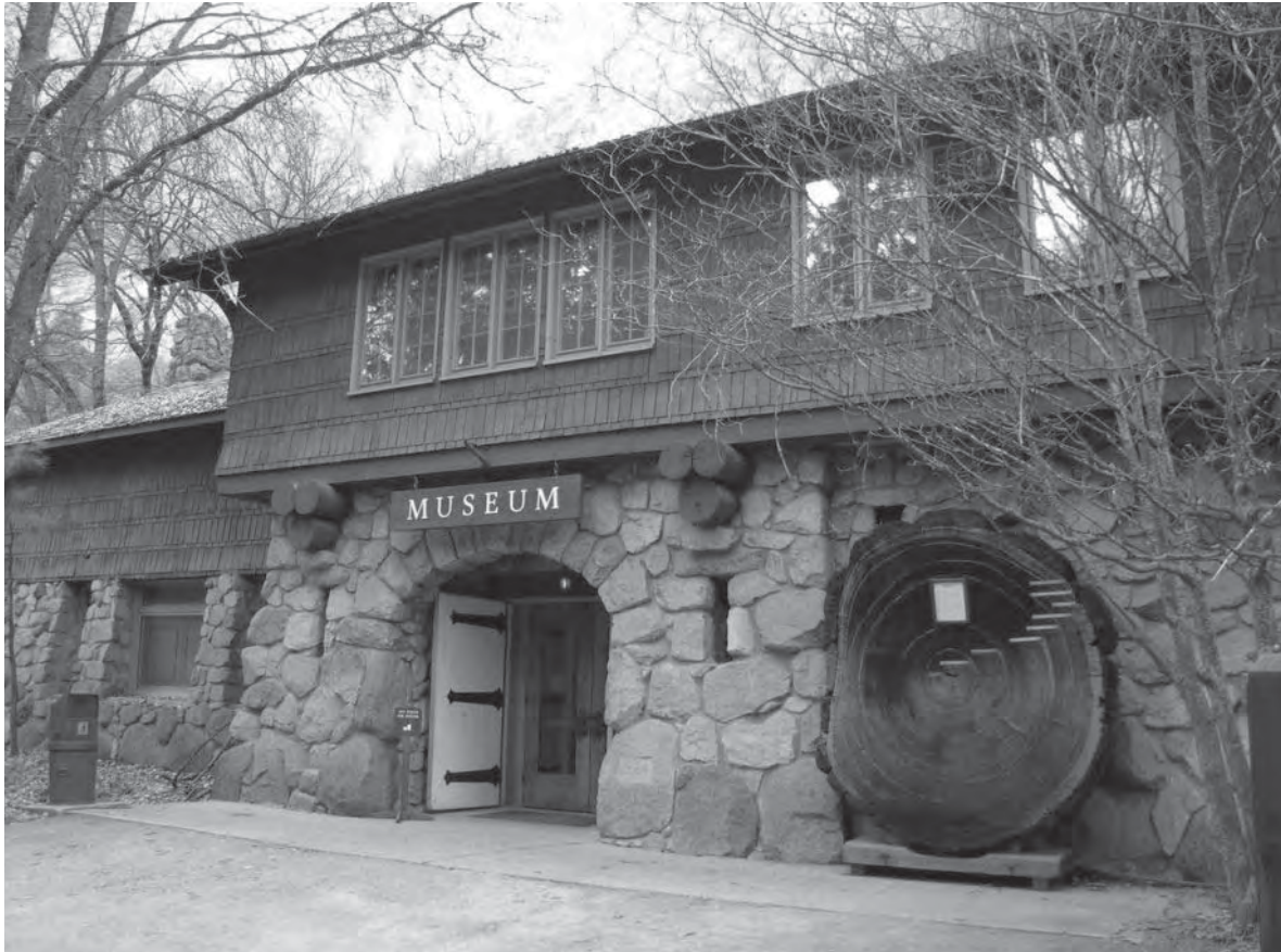
Museum main entrance, south elevation, 2006.
