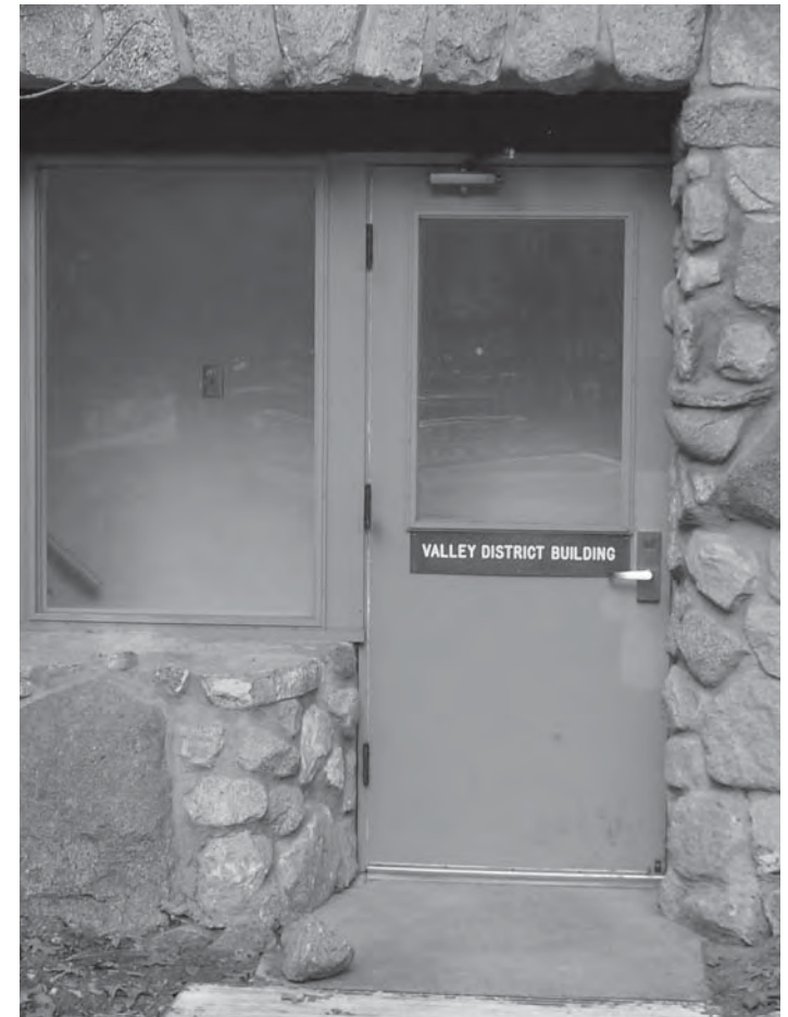
Ranger Entry door at south elevation, 2006.
