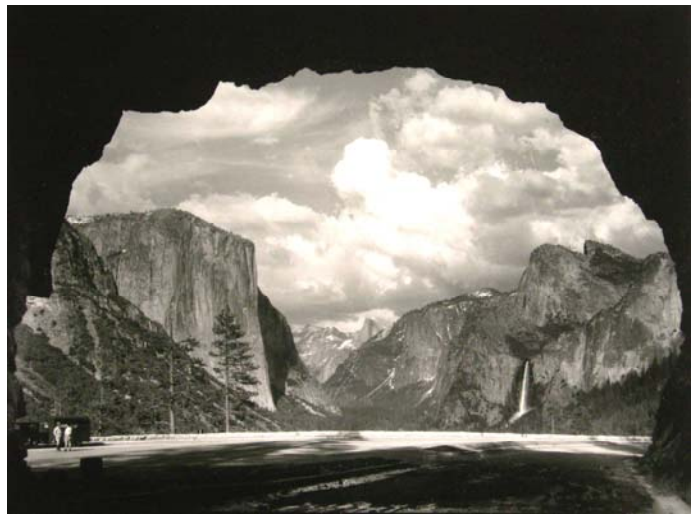
Tunnel View in 1933, after completion of the Wawona Tunnel.
