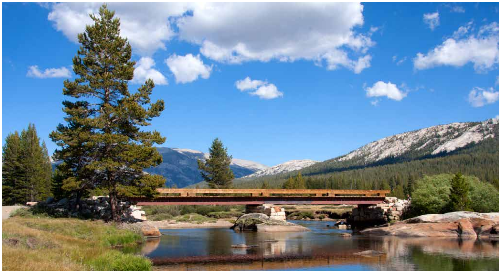
Soda Springs Bridge Photo by Greg Frediani
