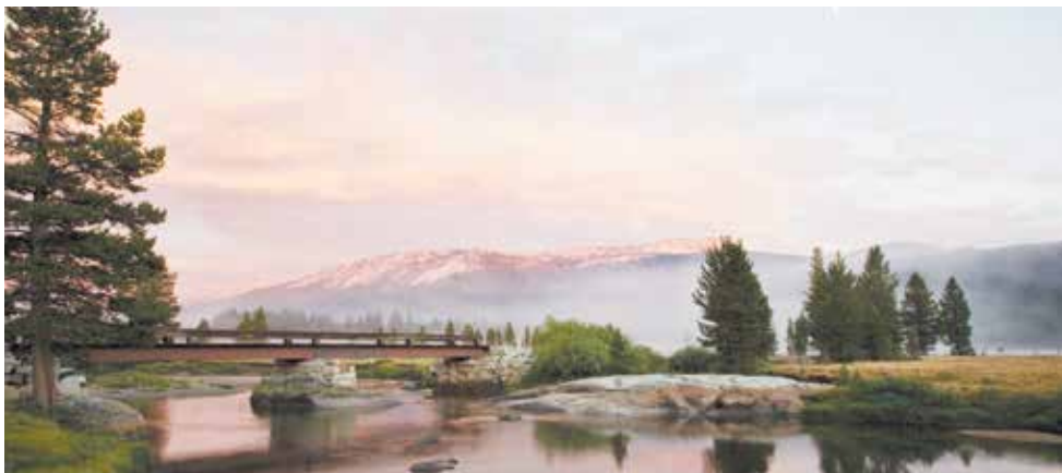
Bridge over the Tuolumne River at Tuolumne Meadows. Photo by John Sun
