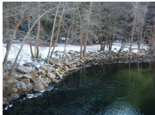
Since the late 1800s, many of Yosemite Valley's rivers and creeks were lined with large stones, called riprap, to prevent the river from widening. Riprap that is no longer functional will be removed or replaced with structures designed to incorporate live plants that will naturally stabilize the bank and enhance riparian habitat. NPS Photo.
