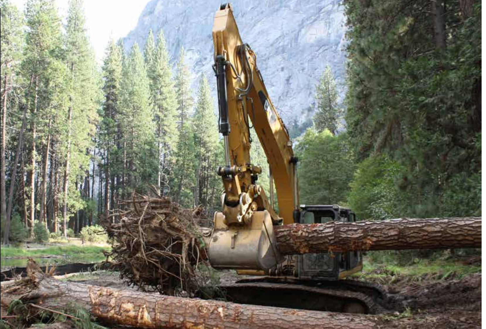
An excavator moves a 60ft tree trunk into position in the river, where it will slow water down and cause sediment to deposit. Read more about restoration efforts along the Merced River on page 10. NPS Photo
