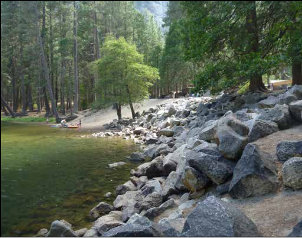
Left: The riverbank at Housekeeping Camp before restoration. Riprap covers the steep banks. Right: The riverbank at Housekeeping Camp two years after restoration. NPS Photos
