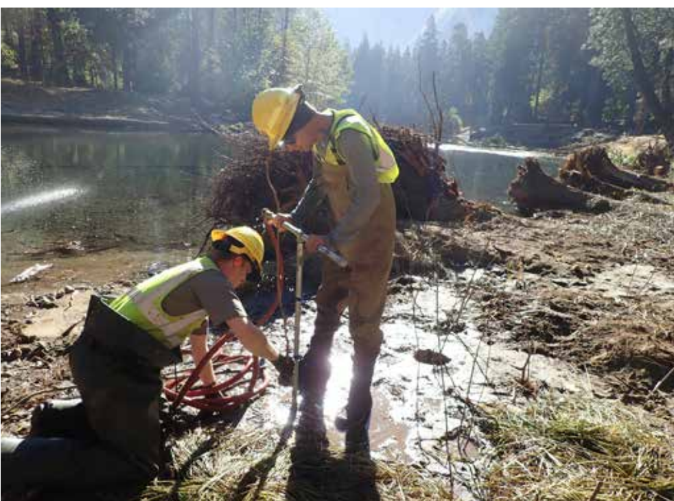
NPS staff plants willow shoots using a high-powered water jet called a hydrodrill. NPS Photos
