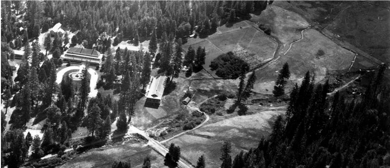
FIGURE 57. AERIAL VIEW OF THE WAWONA HOTEL COMPLEX SHOWING THE ORCHARD CA. 1925 (PHOTO: COURTESY OF TOM BOPP).
