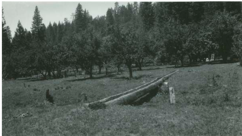
FIGURE 18. A HISTORIC IRRIGATION FLUME IN MCCAULEY ORCHARD, HEWN FROM A LOG.
