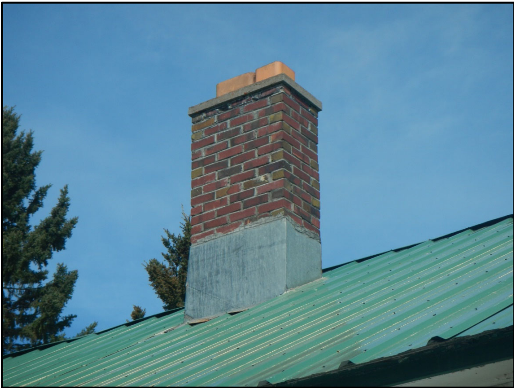
Photograph 6: CAA Quarters, chimney detail
