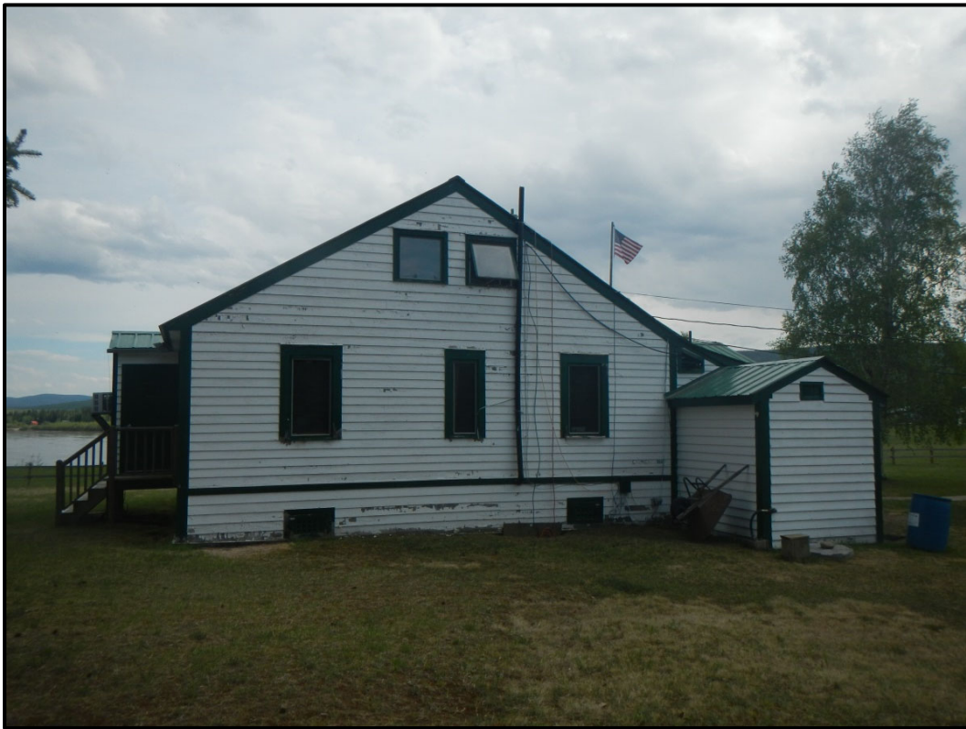
Photograph 4: CAA Quarters (north elevation)
