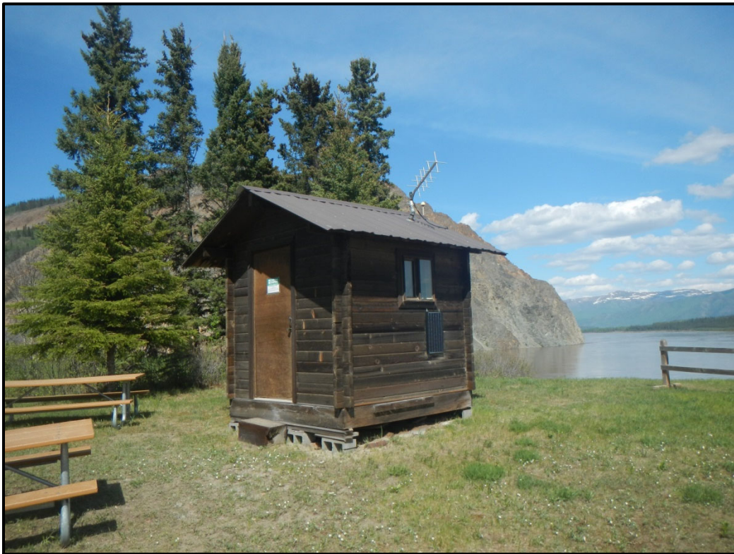
Photograph 8: CAA Quarters outbuilding, USGS Gauging Station
