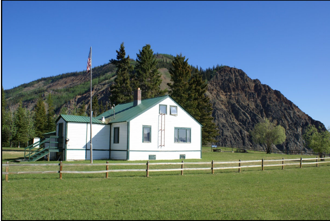
Photograph 1: South elevation of CAA Quarters (Yukon-Charley Rivers Field Office) with Eagle Bluff
