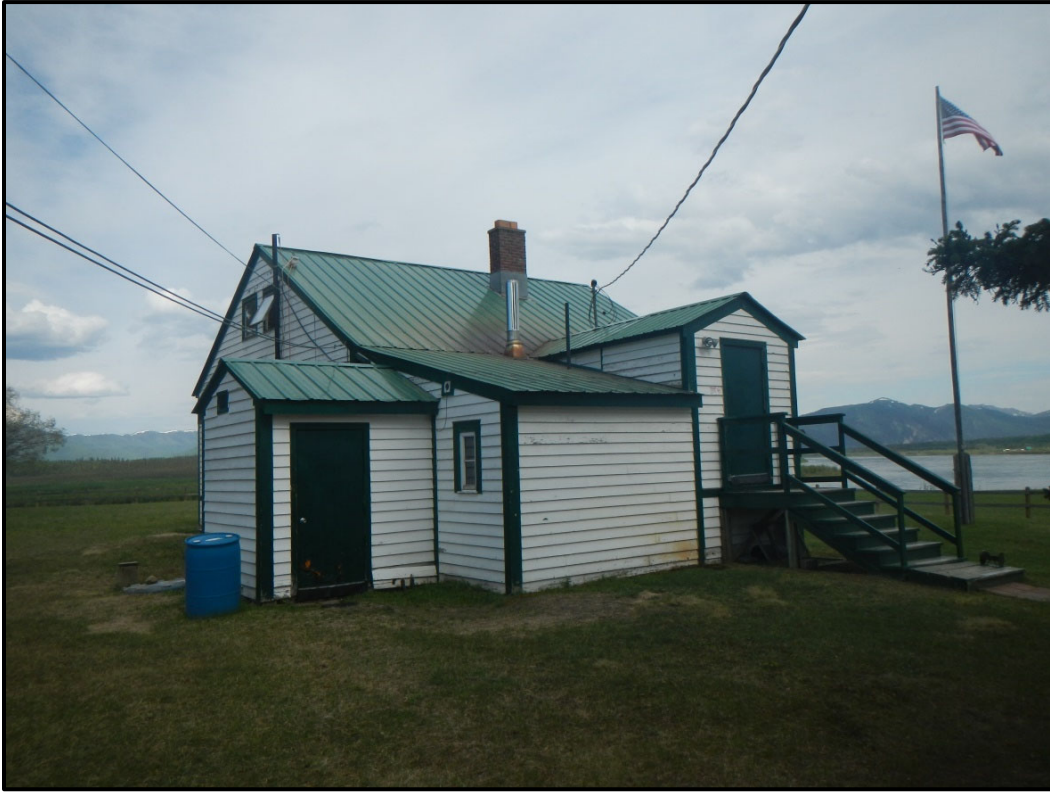
Photograph 5: CAA Quarters with additions (north and west elevations)
