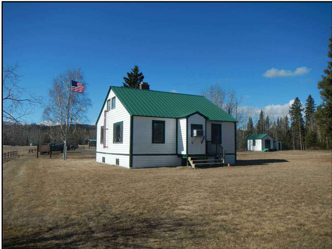
Photograph 2: CAA Quarters (south and east elevations)
