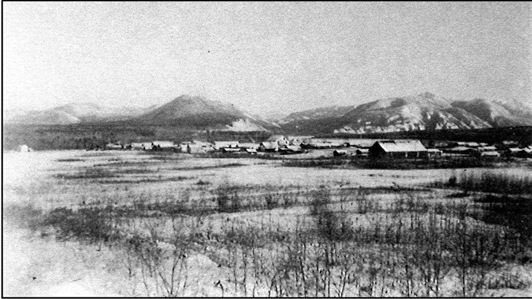
Figure 1: Airstrip in winter with CAA Quarters at far left and Eagle to the right, 1942
