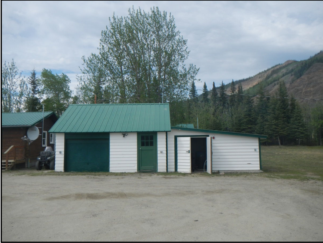
Photograph 9: CAA Quarters outbuildings, garage and shed addition
