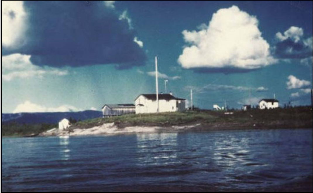
Figure 5: CAA building at Koochak between Kobuk and Shungnak on the Kobuk River, 1951
