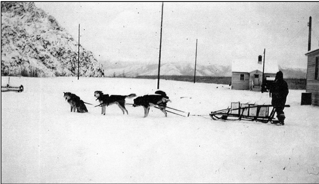
Figure 2: CAA Quarters, newly completed, behind dog team carrying drinking water, 1942
