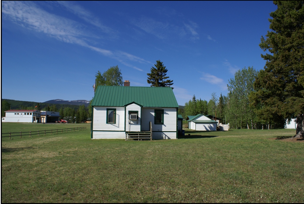
Photograph 3: CAA Quarters (east elevation)
