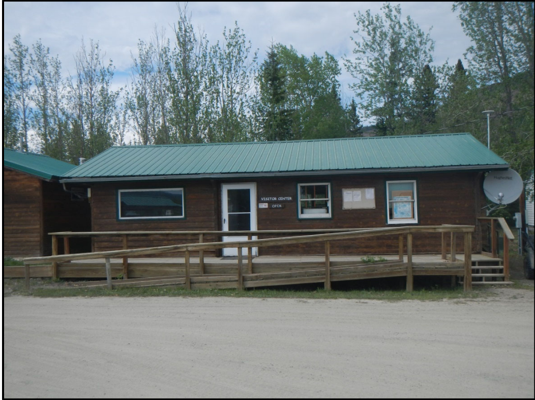
Photograph 10: Yukon-Charley Rivers Visitor Center, adjacent to CAA Quarters
