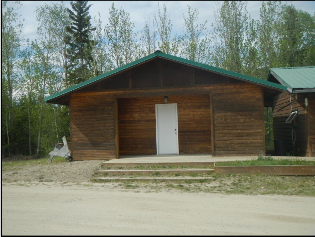
Photograph 11: Yukon-Charley Rivers Visitor Center Public Restrooms, adjacent to CAA Quarters
