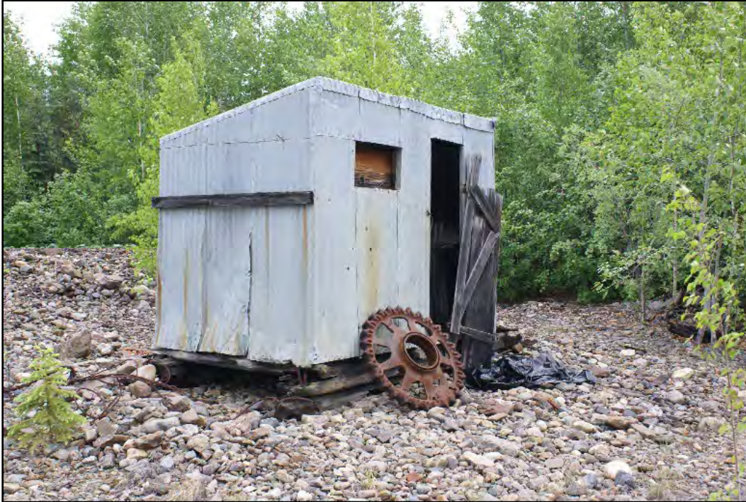
Photograph 5: A wanigan with log skids used to support drilling operations into the 1980s
