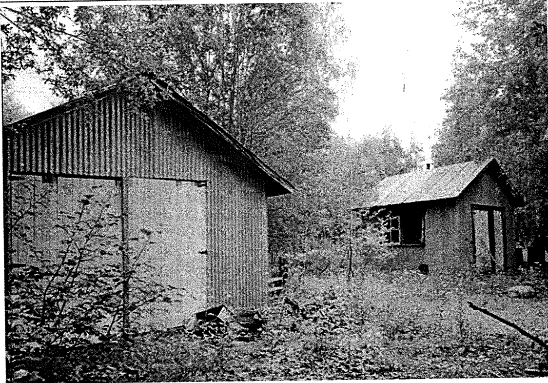
Cheese Creek: Garage/Warehouse and Blacksmith Shop/Storage, 1984; HABS-HAER, 00798pv.
