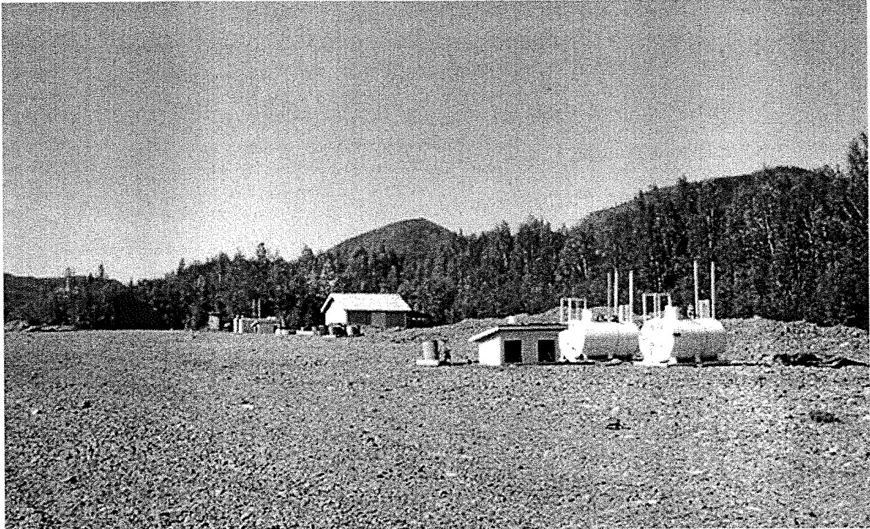
Coal Creek airstrip, 2002; NPS-AKSO Cultural Landscapes Program, 077.
