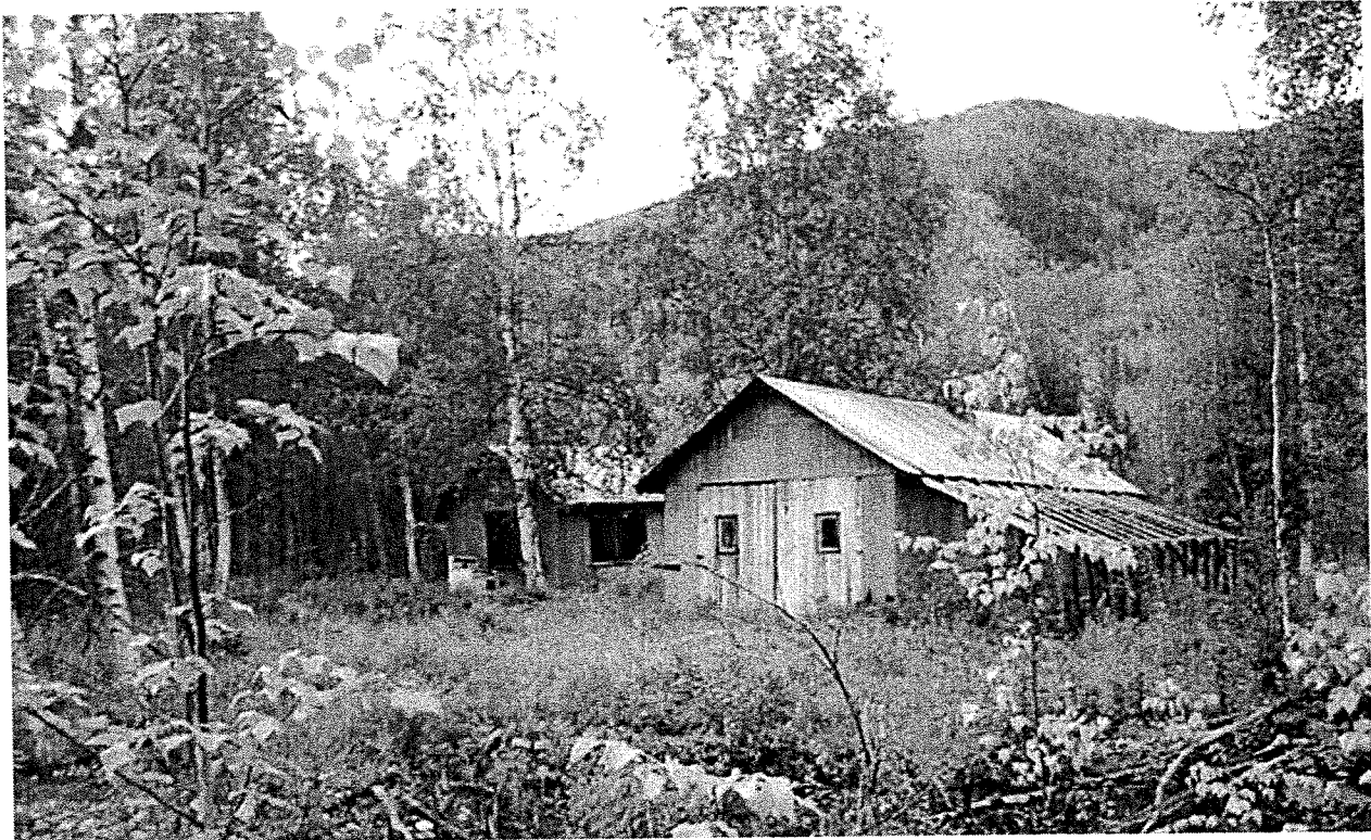
Cheese Creek Blacksmith Shop/Storage and Garage/Warehouse, 2002; NPS-AKSO Cultural Landscapes Program, 125.
