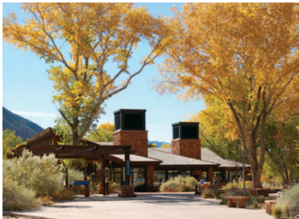
The Zion Canyon Visitor Center is an excellent example of sustainable design.
