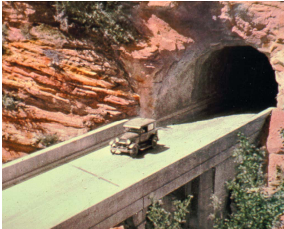
The tunnel was built for cars like this 1930s model.
