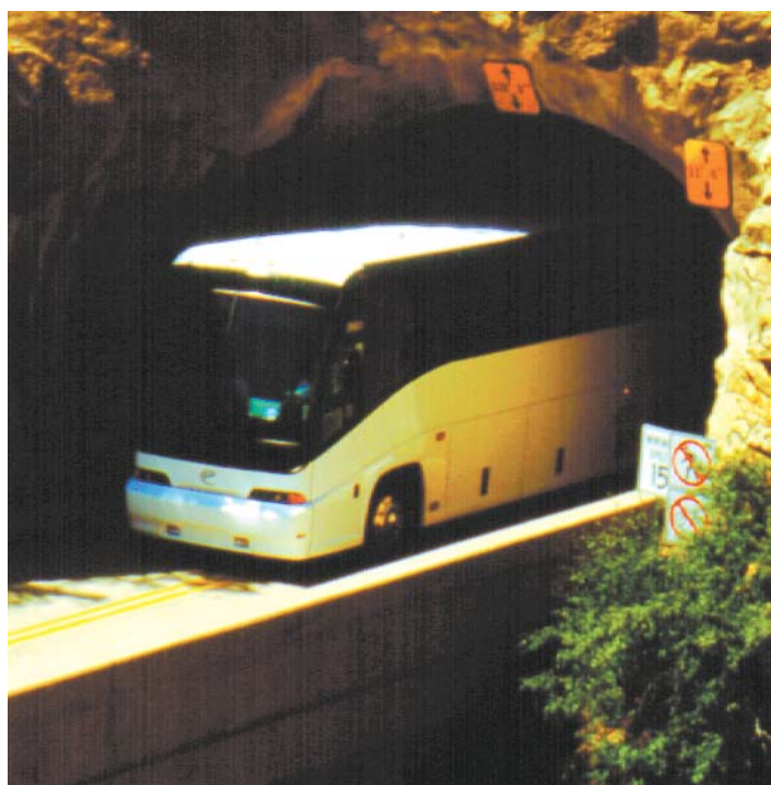
Some modern vehicles require the whole tunnel to themselves.
