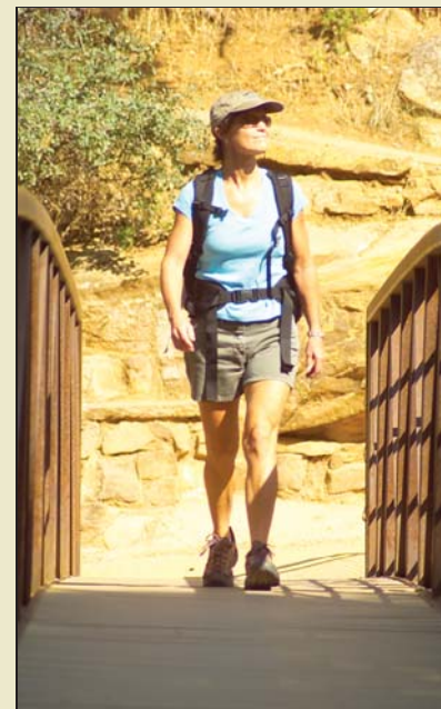
The decks on all the footbridges were replaced with boards made from recycled plastic.
