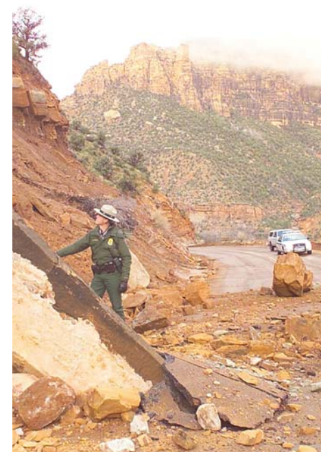
Geology in action; rockfall on the Zion-Mt Carmel Highway switchbacks, February 13, 2005.
