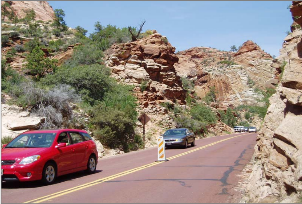
FIGURE 8. ROCK EXPOSURE ON NORTH SIDE OF ROADWAY
