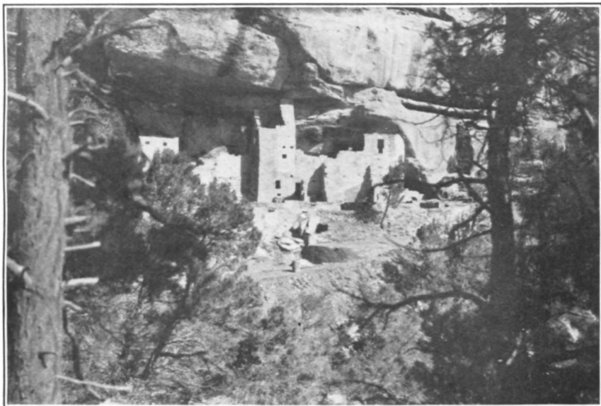
SQUARE TOWER, AFTER REPAIRING
