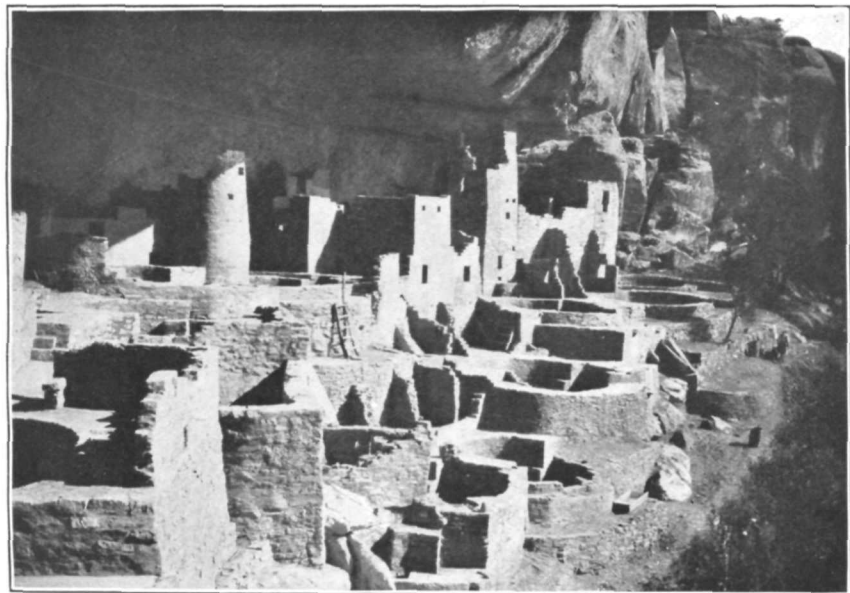
SOUTHERN END, SHOWING REPAIRED TERRACES
