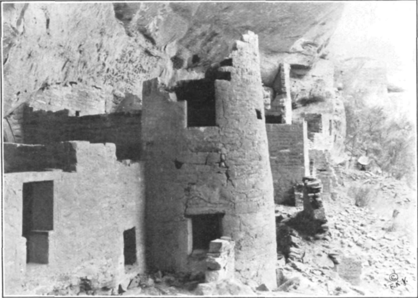
THE ROUND TOWER, FROM THE NORTH
