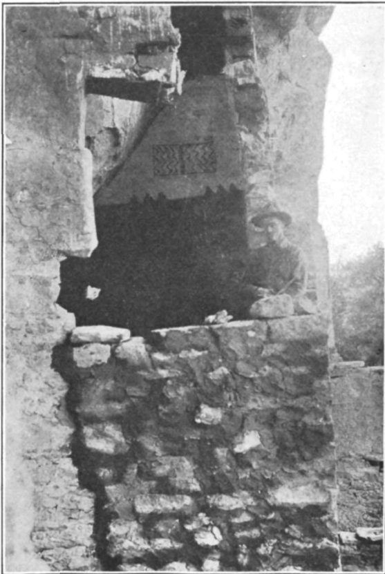
a Third story of square tower, showing dado and decoration
