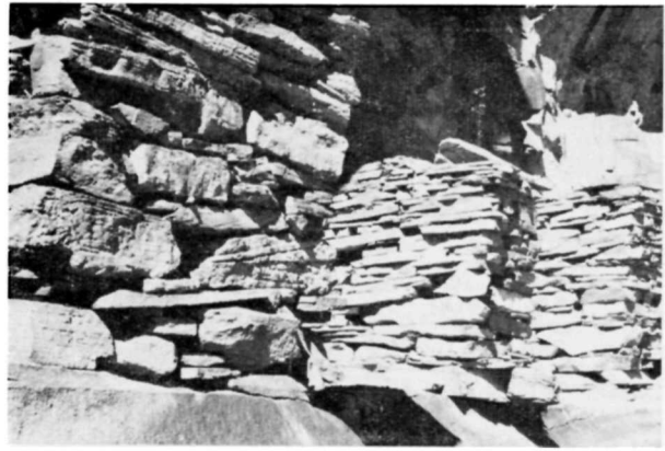
Fig. 31. Construction details of the three masonry columns located at NA3732, Forbidding Canyon.
