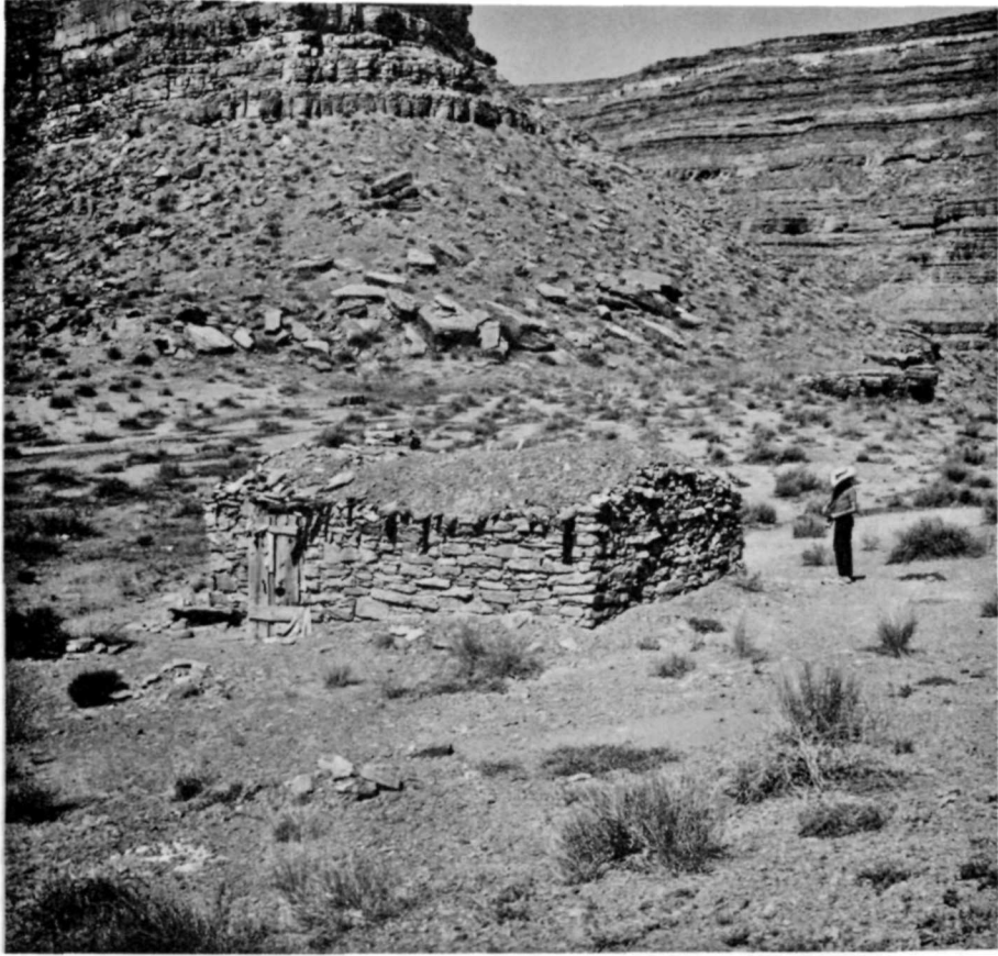
Fig. 5. Mendenhall cabin. Historical site 202.
