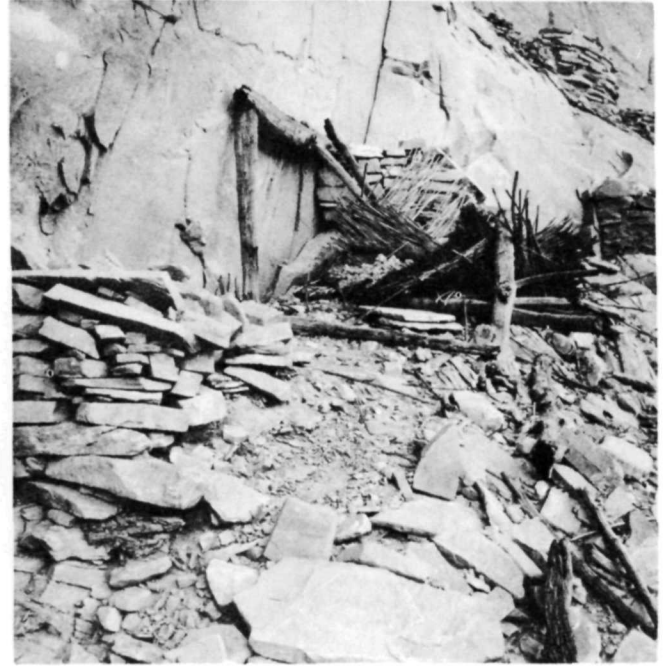
Fig. 6. Collapsed structure, site 42Sa635.
