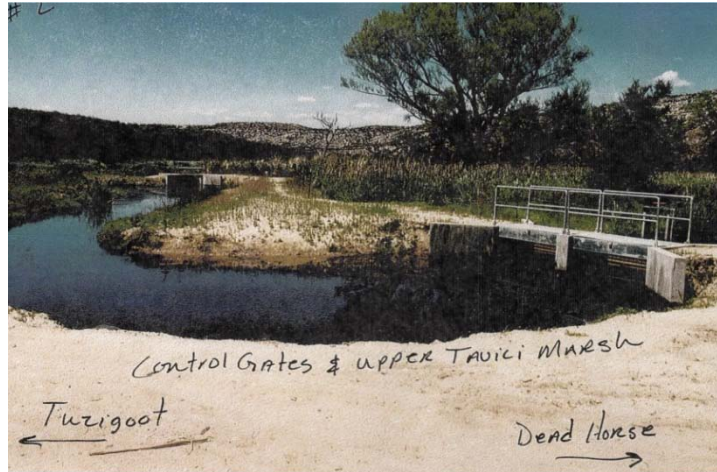
Image 8: Two water control structures installed by the Arizona Game and Fish Department in 1993, as part of the planned restoration of Tavasci Marsh. Courtesy of Tavasci Marsh, FMI.
