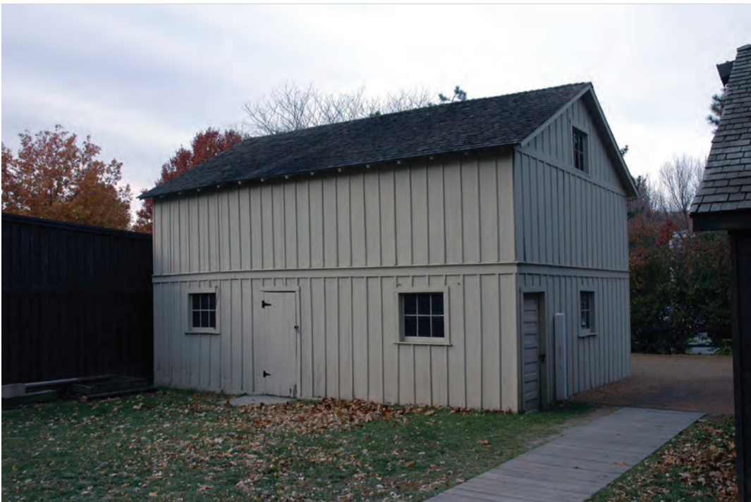
Figure 4. Walter Aitken Barn, 2006.
