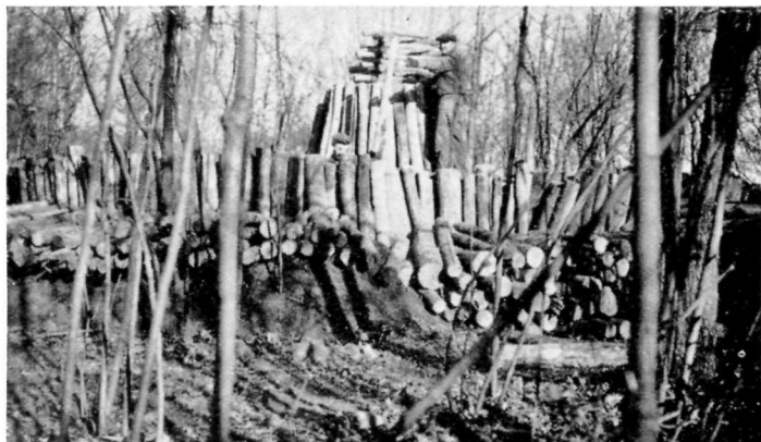
Constructing the chimney
