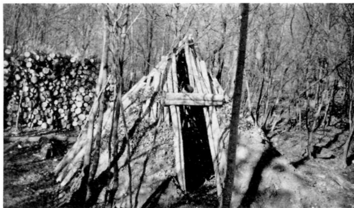
Collier's hut under construction
