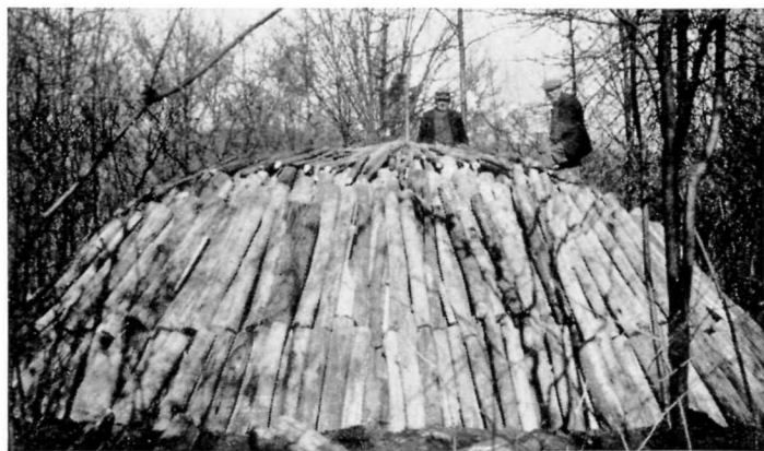
Pit ready for covering
