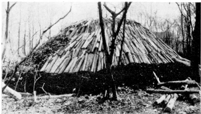
Covering the pit with leaves and dust
