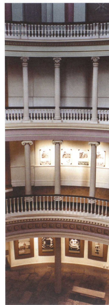
The ornate design of the Old Courthouse rotunda is consistent with the Greek Revival style of 19 th -century public architecture. Each level of columns and balconies becomes progressively more ornamental and complex from the floor toward the top of the dome. (NPS photo)
