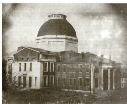
St. Louis County Courthouse in transition, ca. 1850. The early brick courthouse once served as an entranceway and the east wing of the developing courthouse. (Courtesy of Missouri Historical Society)
