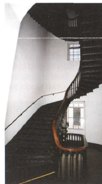
The winding stairway with no middle vertical support was installed and embedded in the walls of the courthouse in 1854. It reflects the prevalent use of cast iron in construction during this era in St. Louis. (NPS photo)
