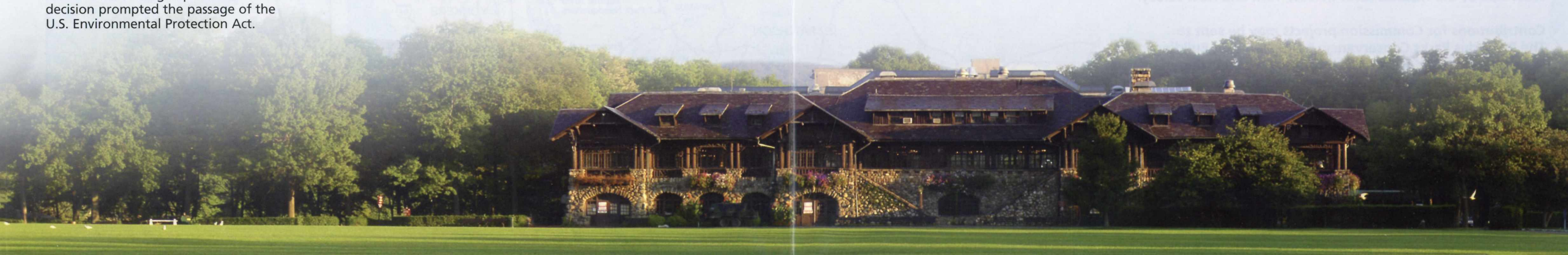
Bear Mountain Inn, built in 1914-15 of local stone and American chestnut trees, set rustic design standards for future park buildings.
