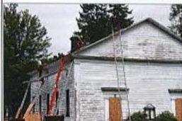
In 2010, workers installed the church's new cedar-shingled roof.
