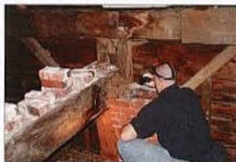
A structural engineer inspects timber deterioration inside the church, 2010.
