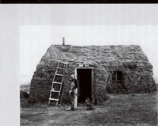
Blocks of sod cut from the deep topsoil of the grasslands were used by settlers to build temporary homes on the treeless plains of America's heartland. These "soddies" offered shelter from the intense heat or bitter cold until lumber could be imported from the
