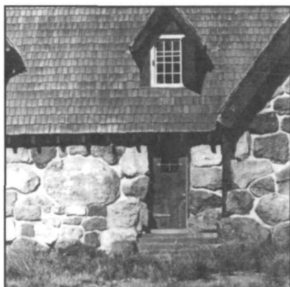
Front entrance of Superintendent's Residence. Note large boulder near door.
