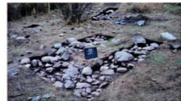
ABOVE: Potential rock fall from what may have been a foundation.
