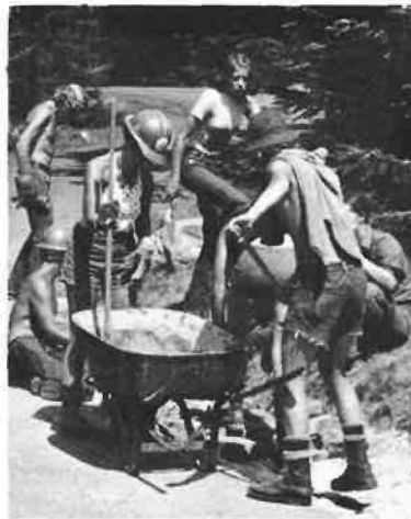
YCC members at Acadia NP mix cement as they prepare to fill an empty roadside ditch.
