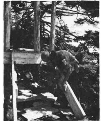
Crew leader completing the final steps of a wooden staircase at Bass Harbor, Acadia NP.
