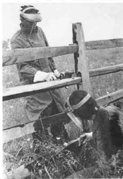
Completing fence project with application of creosote, Harpers Ferry.
