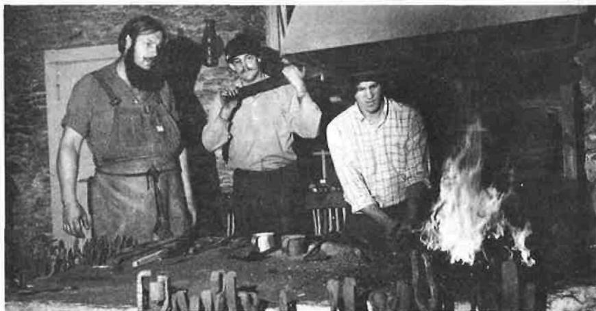
Blacksmith Arnold Schofield, left, researched and constructed the forge he uses to instruct assistants in the building and maintaining of a proper fire.
