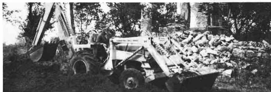
Harold May, heavy-equipment operator, churns the soil beside St. George's Chapel, an on-going preservation project.
