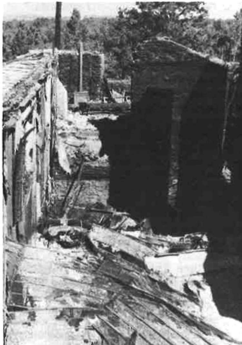
At Navajo National Monument, Ariz., this building was demolished by an explosion of Liquid Petroleum Gas.
