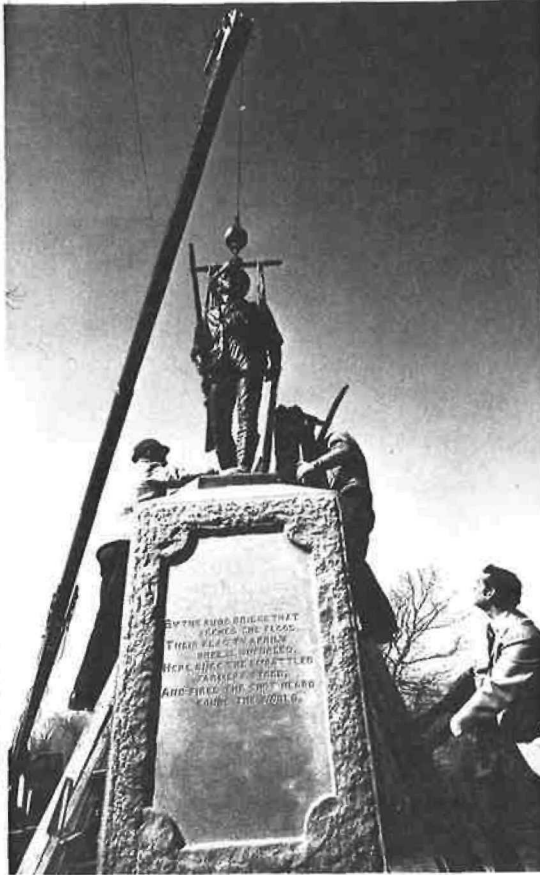
Daniel Chester French's famous statue of the "Minute Man" is hoisted by crane back to its pedestal at North Bridge in Minute Man National Historical Park, Concord, Mass. Holding the ladder for the workers is David Moffitt, superintendent of the park.
