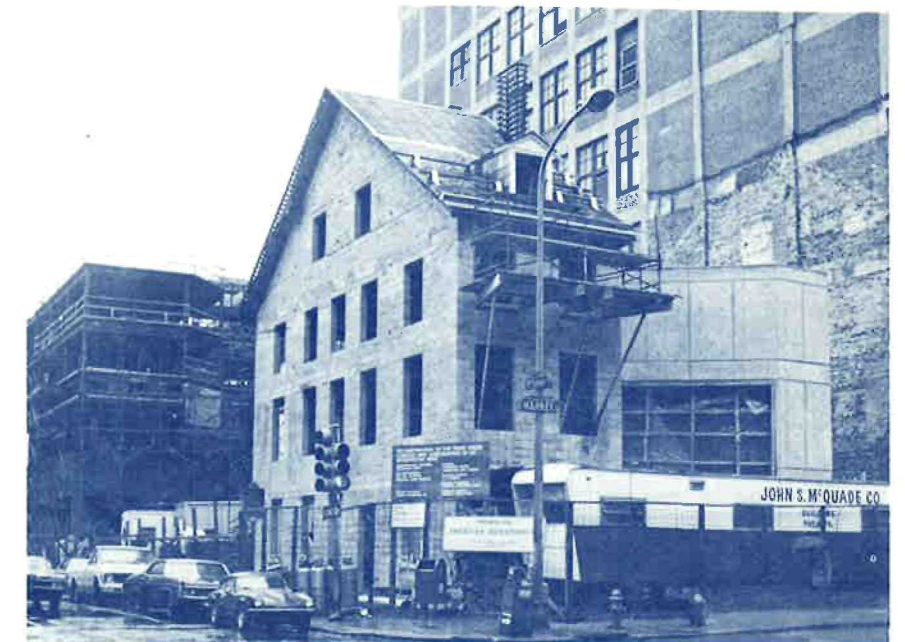
Under construction is Graff House at Independence NMP, Pa. Here Thomas Jefferson drafted the Declaration of Independence in June 1776.
