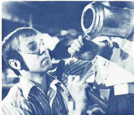
Following casting of cannon, considerable hand work is required to finish ornamental relief designs.
