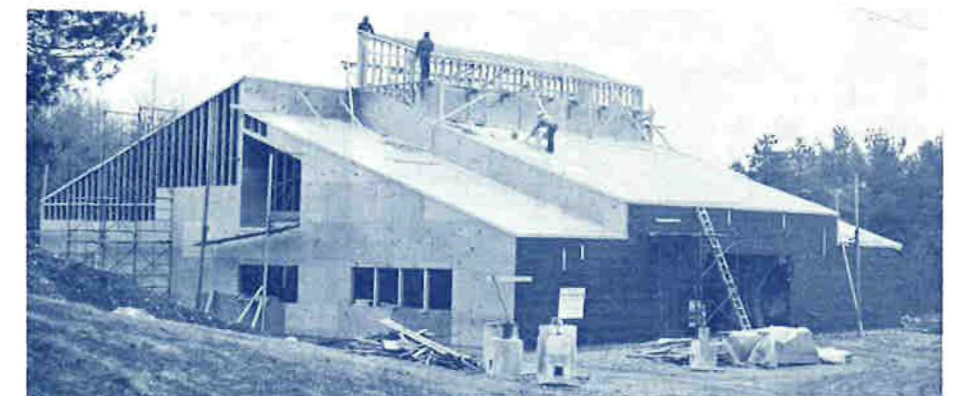
A new visitor center to house exhibits and audiovisual programs is under construction at Minute Man NHP, Mass.
