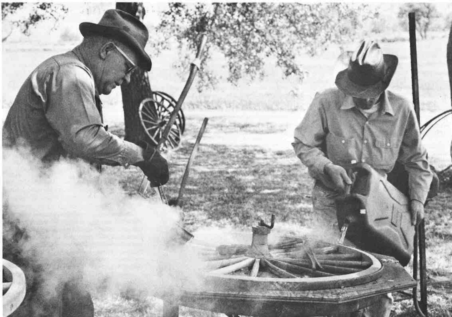
Steam rises as Mel DeWitt, left, and his son, Wayne, pour water on a red-hot wagon tire. After heating in a forge, the expanded tire can be slipped over the wheel. The water cools the tire, causing contraction and cinching the wheel tight.
