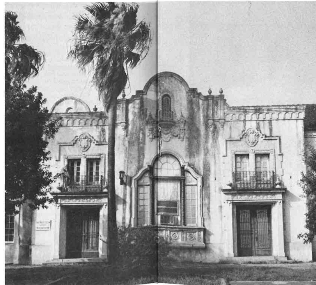
A prime candidate for adaptive reuse, the Southern Pacific Railroad Station in Brownsville is presently slated to become the city's new police department headquarters. photo by: John White.
