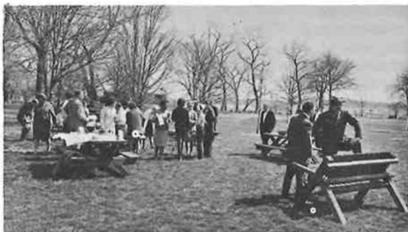
NPS Photo by W. H. Spradley
