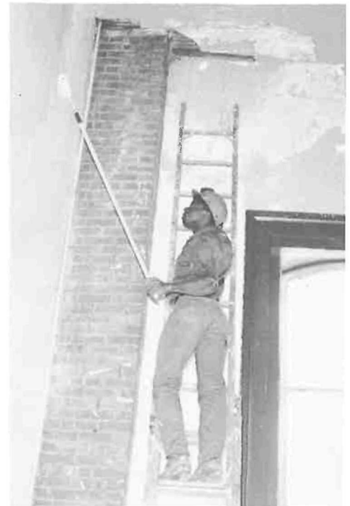
Renovating an historic building
