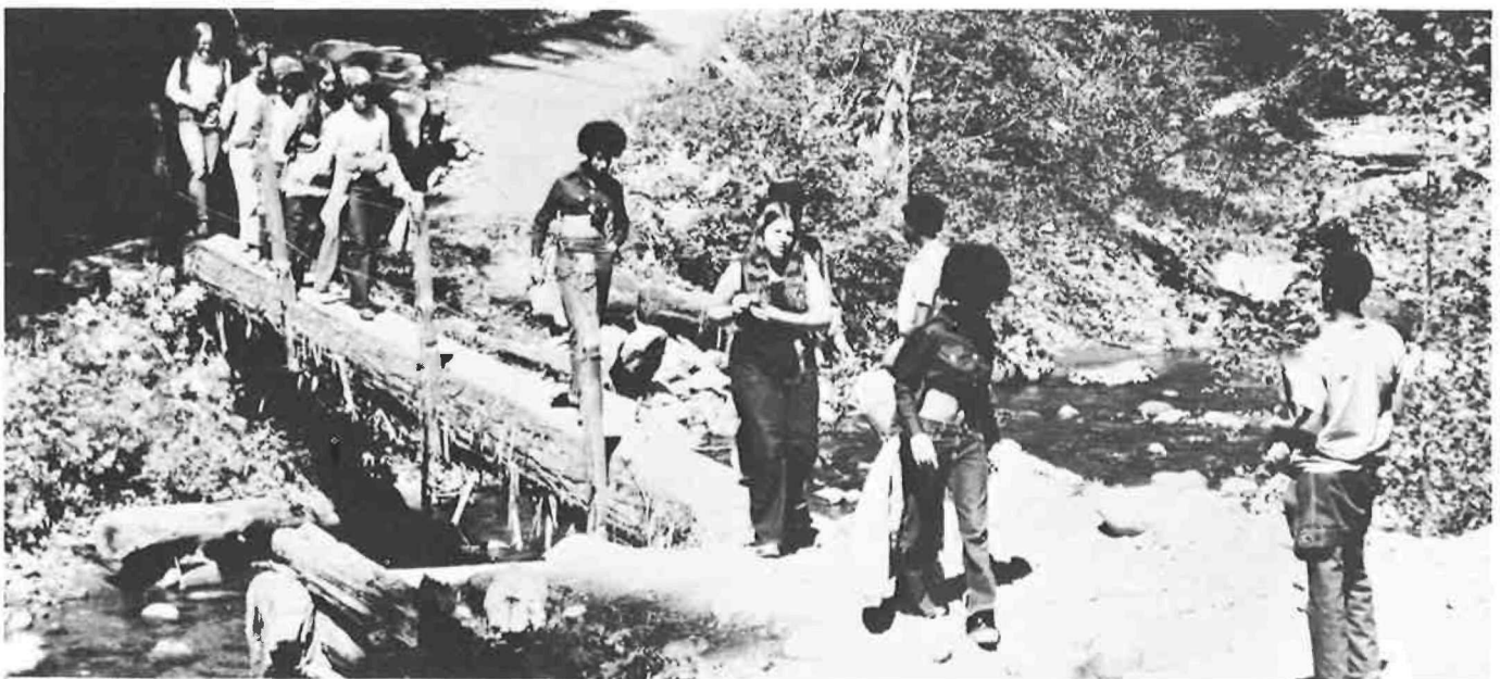
Testing a newly completed footbridge
