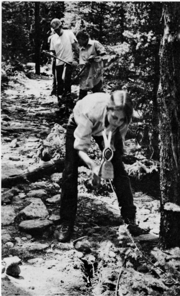
SWINGING A HOEDAG is hard work in rocky soil where these YCCers are digging several miles of shallow trench and burying the Longs Peak emergency telephone line (visible in foreground) which now will be out of sight.
