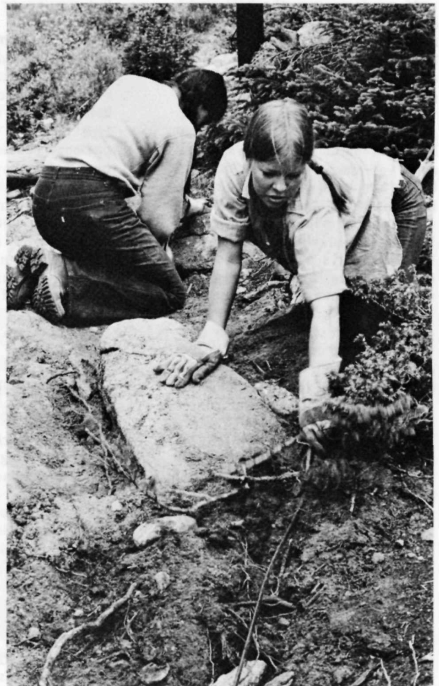
"EXTERIOR DECORATORS" cover the telephone cable with dirt, then camouflage with rocks and logs to erase the scars. They follow the hoedag crew and leave little trace of where the line is buried.
