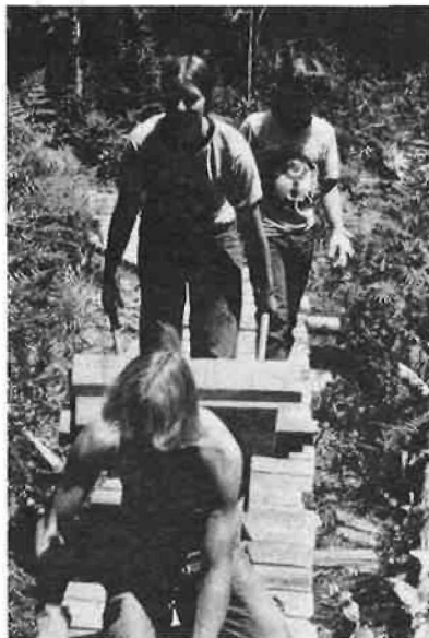
YCC enrollees construct a cedar walk near Lake Ozette in Olympic NP this summer.
