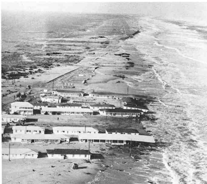
A MID-WINTER STORM the weekend of Feb. 10-11 left motel units and private dwellings near Cape Hatteras National Seashore almost in the ocean. The "protective" barrier dune was completely wiped out at this spot about one mile north of Cape Hatteras Lighthouse, allowing the sea to directly attack the developed area.
