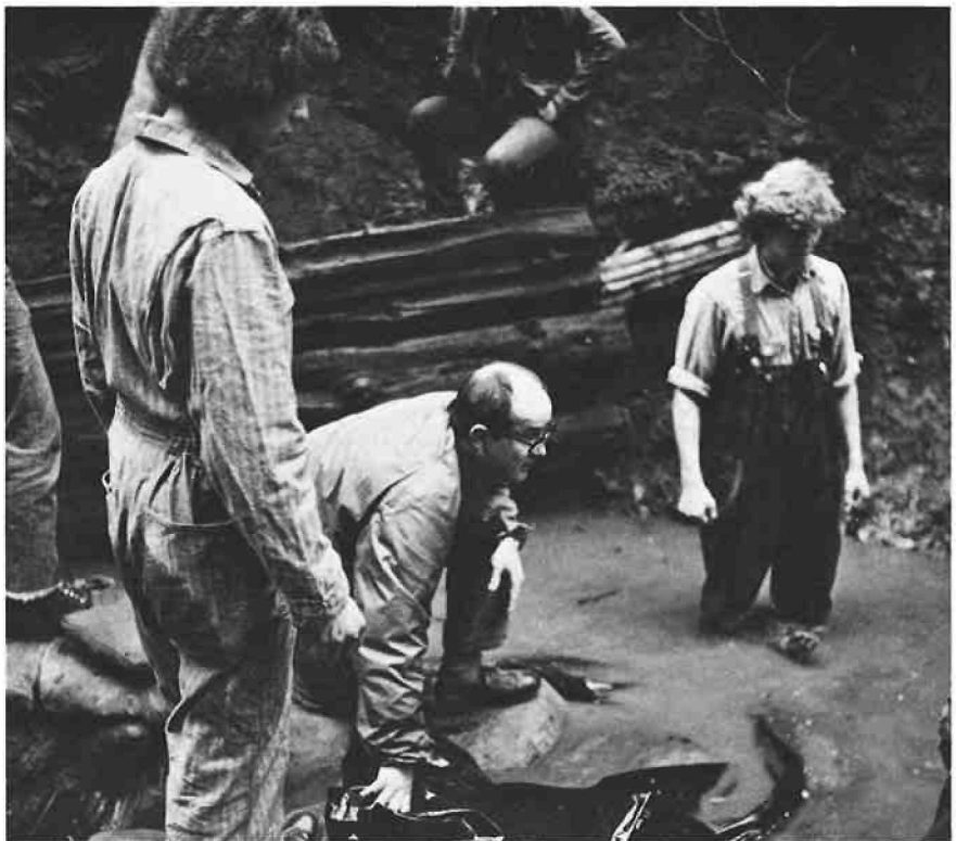
BRUCE WEBSTER AND HIS CLASS build a cofferdam across a creek to protect a water pipe from damage during heavy rainfall. The plastic is used to divert the creek while concrete hardens. The group spent 560 hours to construct the dam.
