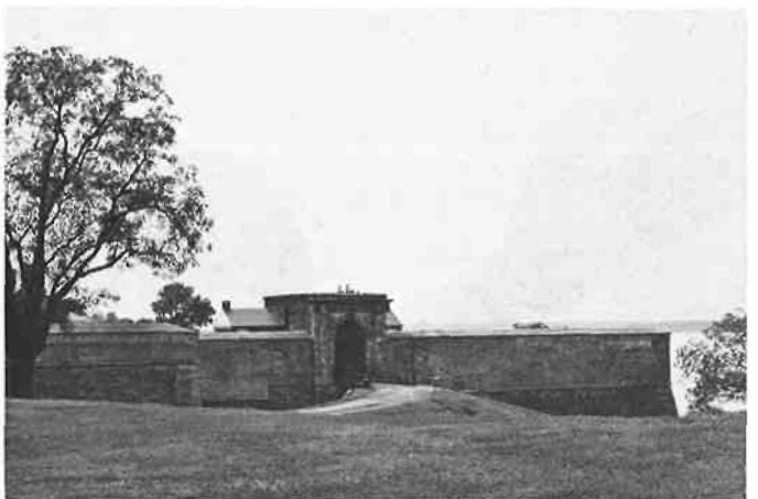
The main entrance to Fort Washington. The gateway is entered over a dry moat.
