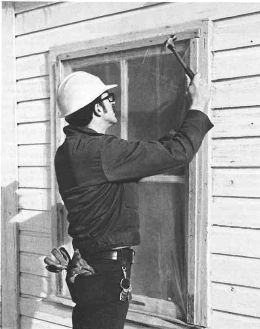
Clear plastic sheeting was placed over the windows of all shops, office buildings, and many residences to prevent the escape of heat.
