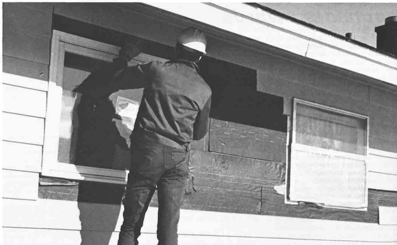
Metal window frames were replaced with wooden frames to prevent loss of heat through conduction.
