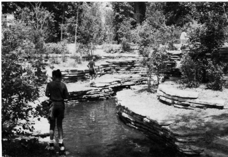
Fig. 2. Recent rehabilitation work in Columbus Park included the waterfall, cascades, rocky brook and associated landscape for this popular Prairie feature in Jens Jensen's most extant and authenticated park in Chicago. Photo by the author.
