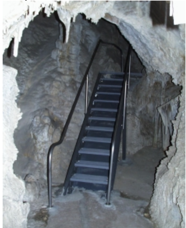
One of the recently constructed stairways. (NPS Photo by Jon Jasper)
