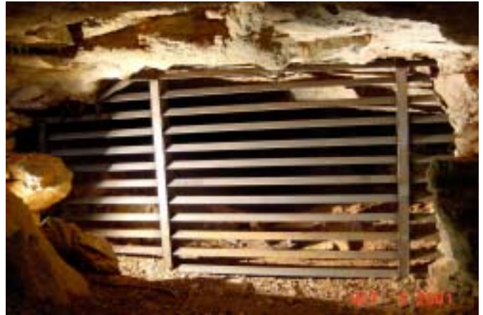
Completed bat gate, Capps Mine portal #2. (NPS photo by Chuck Bitting)
